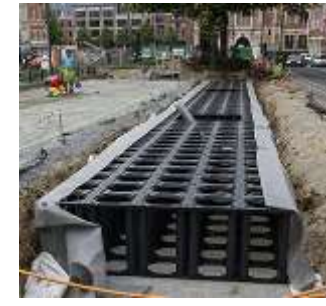
NL: structural Soil cell + bioretention
